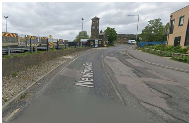
Newtown Road Approach from North-East Direction – Google
